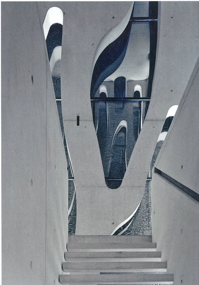
1 Betonguß in fünf Etappen Concrete cast in five layers
